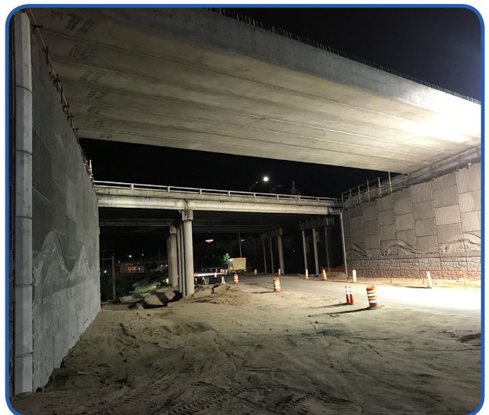
Cranes setting girders on Gruma Street bridge
