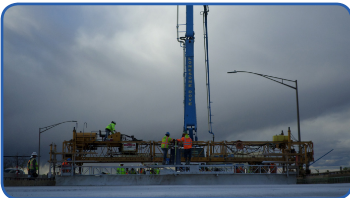
Paving northbound bridge at Indiana Avenue
